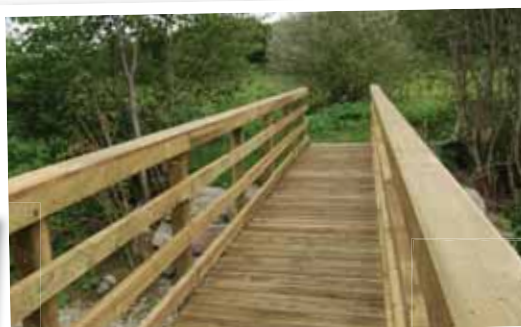
New bridge at Cultullich
